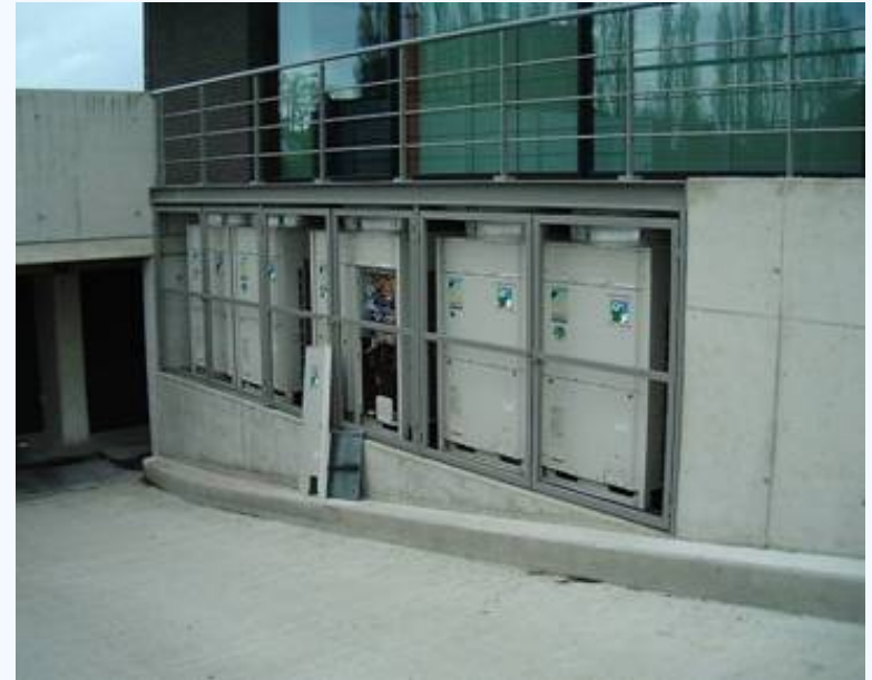
Unable to do maintenance on this unit
