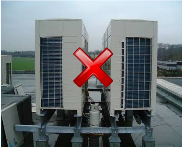
Not enough space for maintenance
